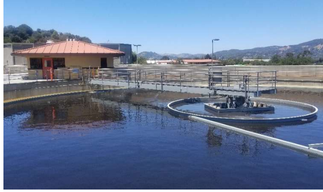
Secondary clarifier in operation
