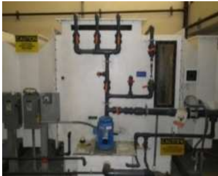
Solids Handling Building odor control scrubber
