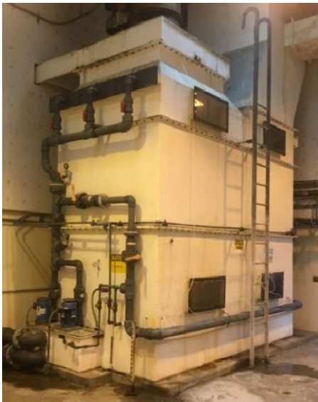
Headworks odor control scrubber
