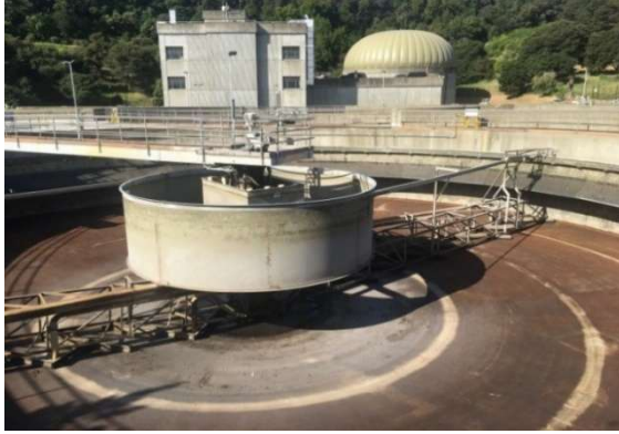
Secondary clarifier internal equipment
