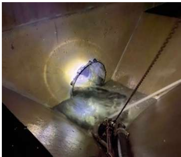
48" Primary Effluent Pipe – Interior
