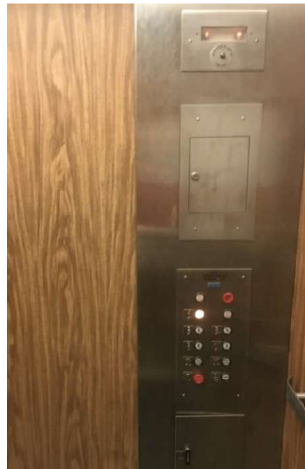
Elevator Control Panel
